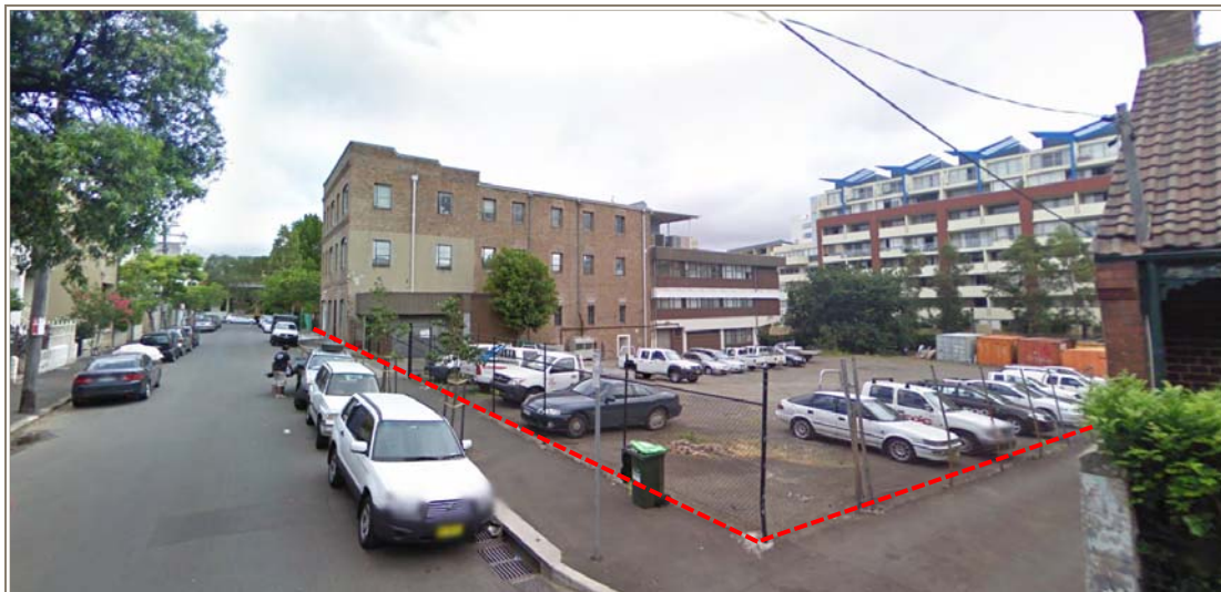
Figure 2: View south, down Junction Street, along the site's eastern boundary
